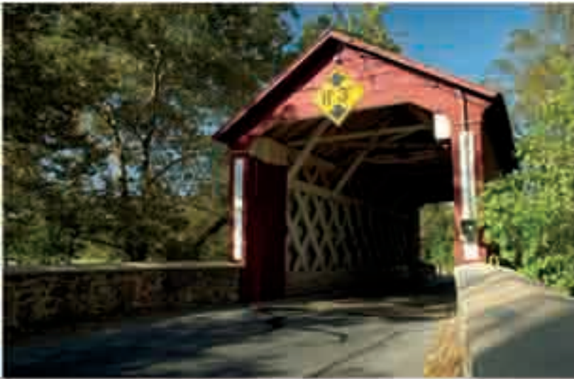
5. Brackenville Road (Ashland Bridge)
