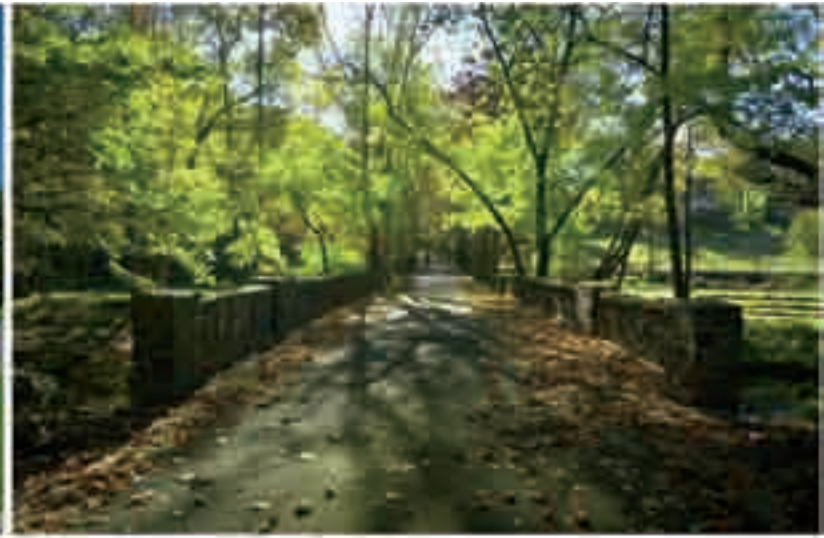
30. Creek Road Bridge
