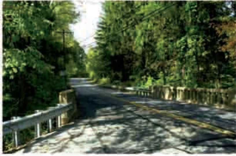
18. Barley Mill Road at Rolling Mill Road
