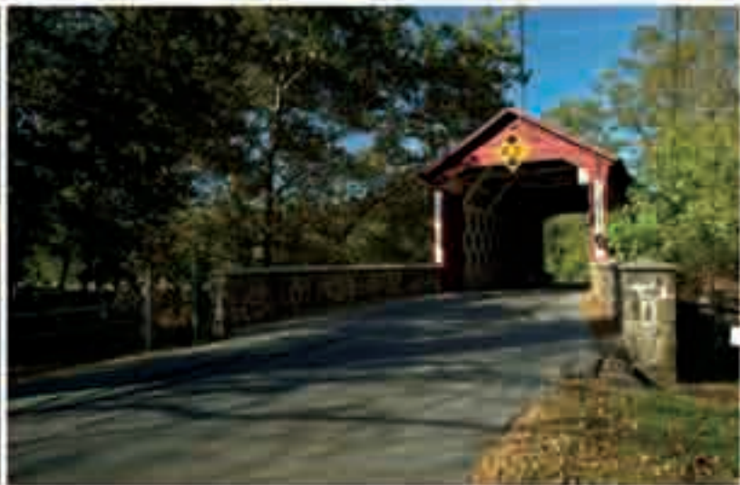
4. Brackenville Road (Ashland Bridge)
