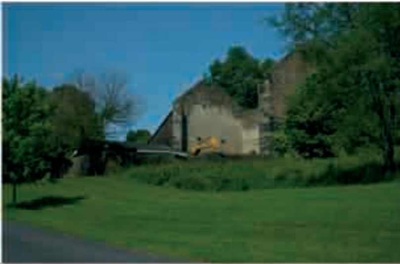
69. Creek Road (Yorklyn Stone Barn Ruin)
