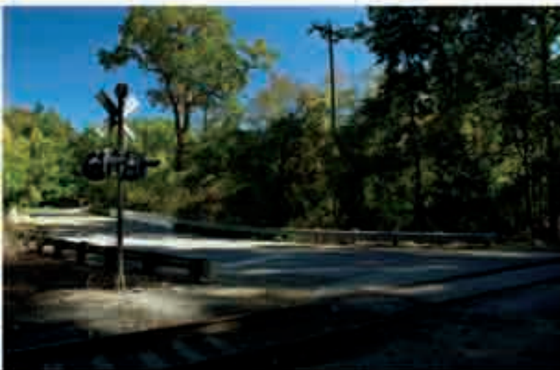
39. Mt. Cuba Road railroad crossing
